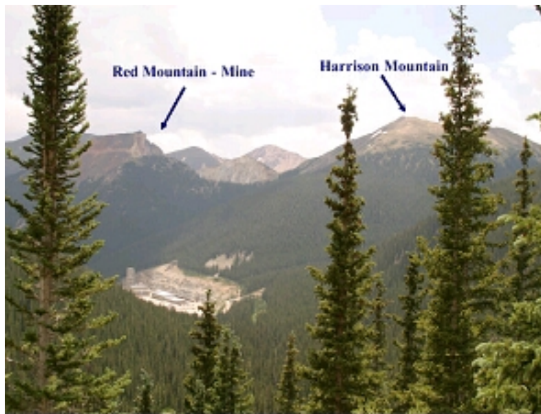
Figure H1. View of the Henderson Mine site showing mine buildings, Red Mountain mining area, and Harrison Mountain.
